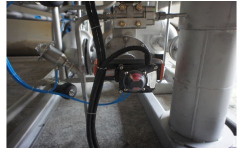
风动换向装置 Pneumatic Flow Reverse Device
